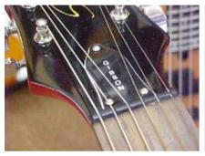
On many guitars you will find the truss rod nut located underneath a cover on the head stock of your neck
